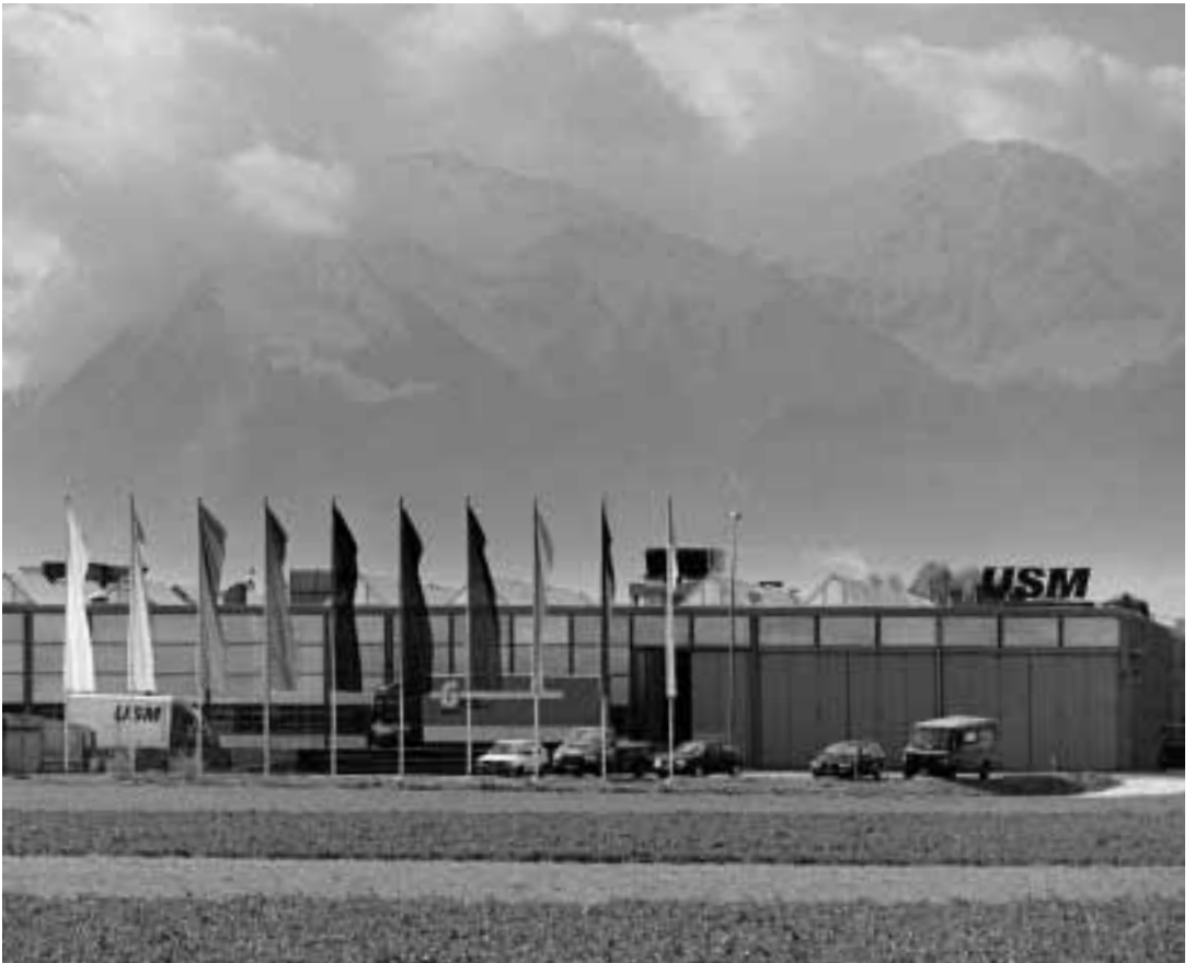
Factory building in Munsingen, Switzerland
